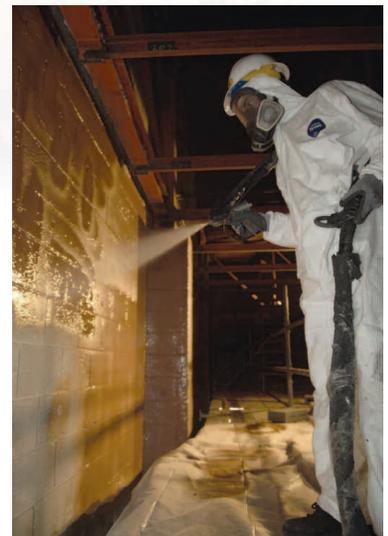
**Figure 1. An Anti-Terrorism Bomb Blast Protective Coating is sprayed onto the Interior Walls of an Air Force Base facility. (Photo taken by Airman 1st Class Nicholas Pilch and provided courtesy of the US Air Force)**
